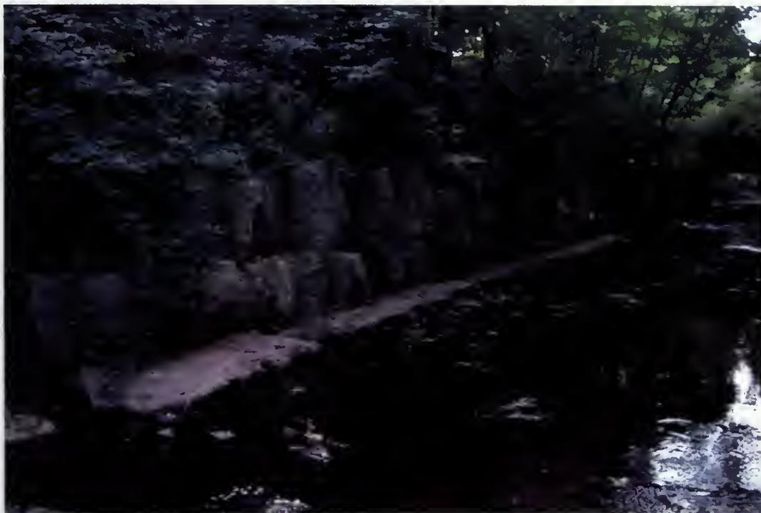
**Figure 3.6** Armourstone wall along Appleby Creek Burlington, Ontario. The wall is protecting residential property. The creek flows from right to left.
