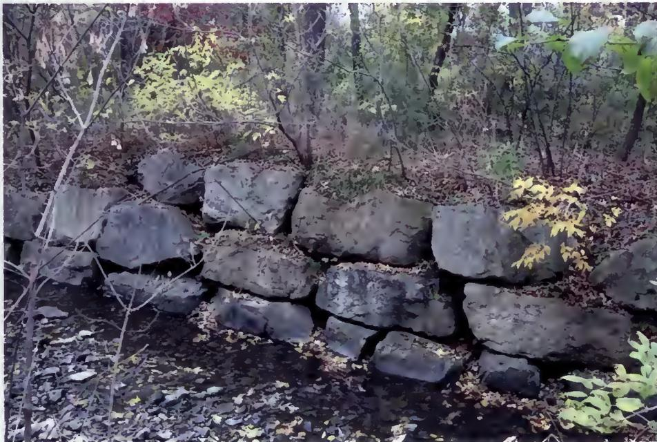
**Figure 6.2** Section of Loyalist Creek, Mississauga, Ontario. The stones used in armourstone walls are of variable shapes and sizes which lead to the presence of large gaps.
