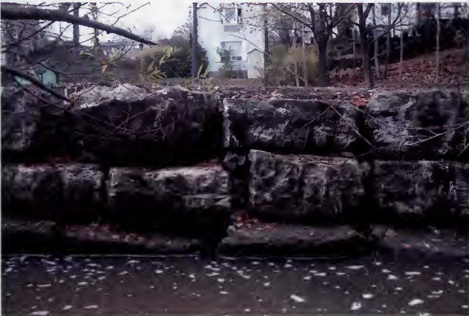
**Figure 6.4** Forty Mile Creek Grimsby, Ontario. Riprap (small stones) is used in between the armourstone blocks to fill in the gaps.
