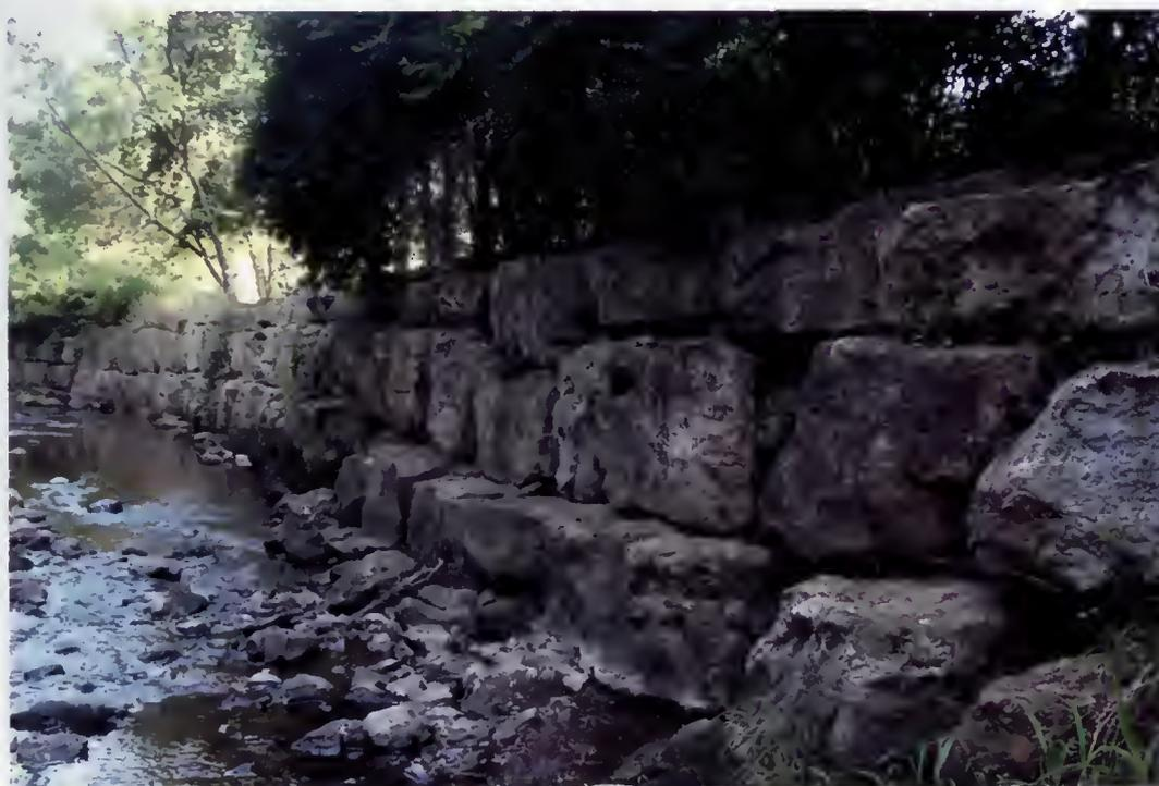
**Figure 3.5** Armourstone wall along Tuck Creek Burlington, Ontario. The right side of the photo is residential property. Photo is looking downstream.
