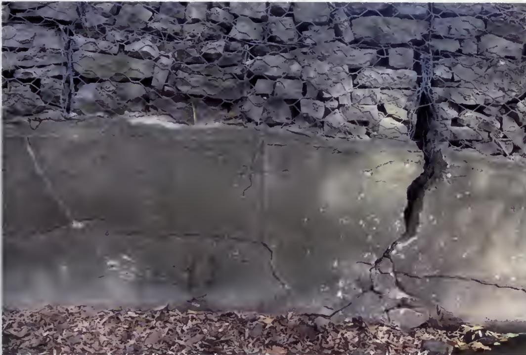
**Figure 2.1** A concrete wall along Forty Mile Creek in Grimsby, Ontario. A large crack running down the wall can be noticed, which is also forcing the gabion basket on top of the wall to be pulled apart.
