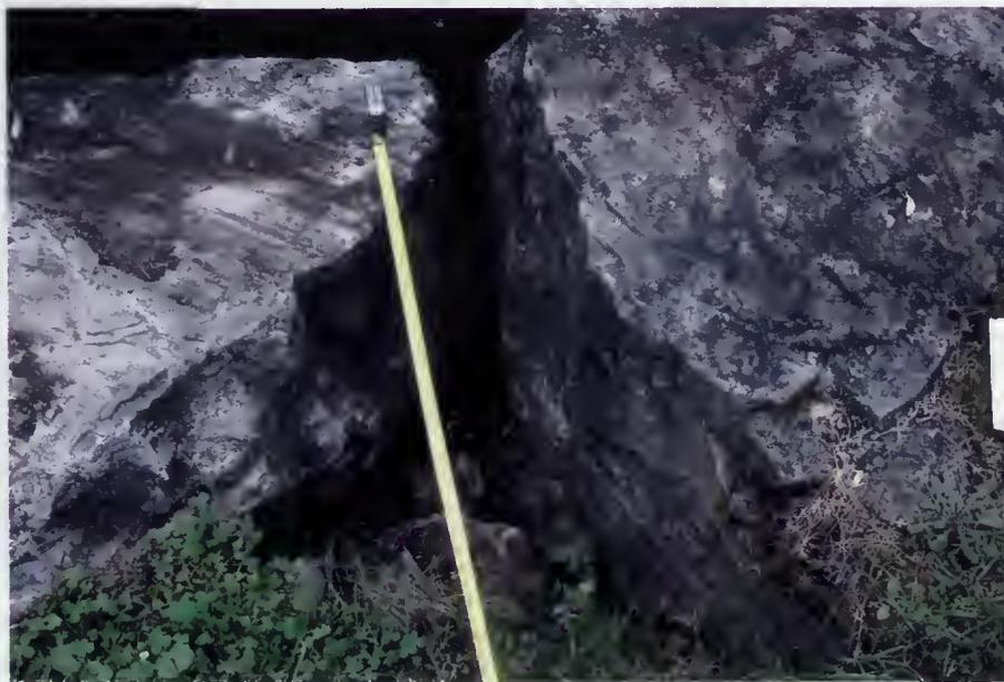
**Figure 5.3** One of the gaps measured between the armourstones along the wall at Forty Mile Creek, Grimsby. This gap was measured as a triangular prism.
