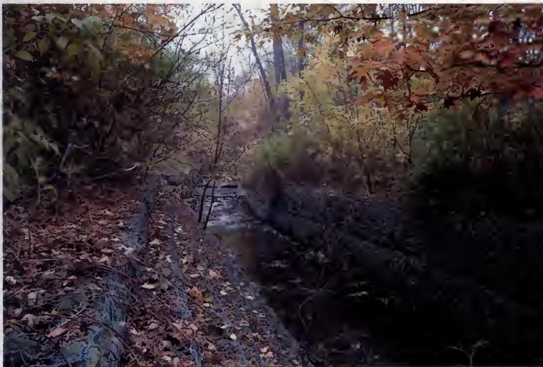
**Figure 2.2** Gabion baskets lining a section of the bank along Loyalist Creek, Mississauga, Ontario. Photo is looking upstream. On the left hand side of the photo the gabion baskets are lining the bank adjacent to a public trail; on the right hand side the gabion baskets are protecting residential property.
