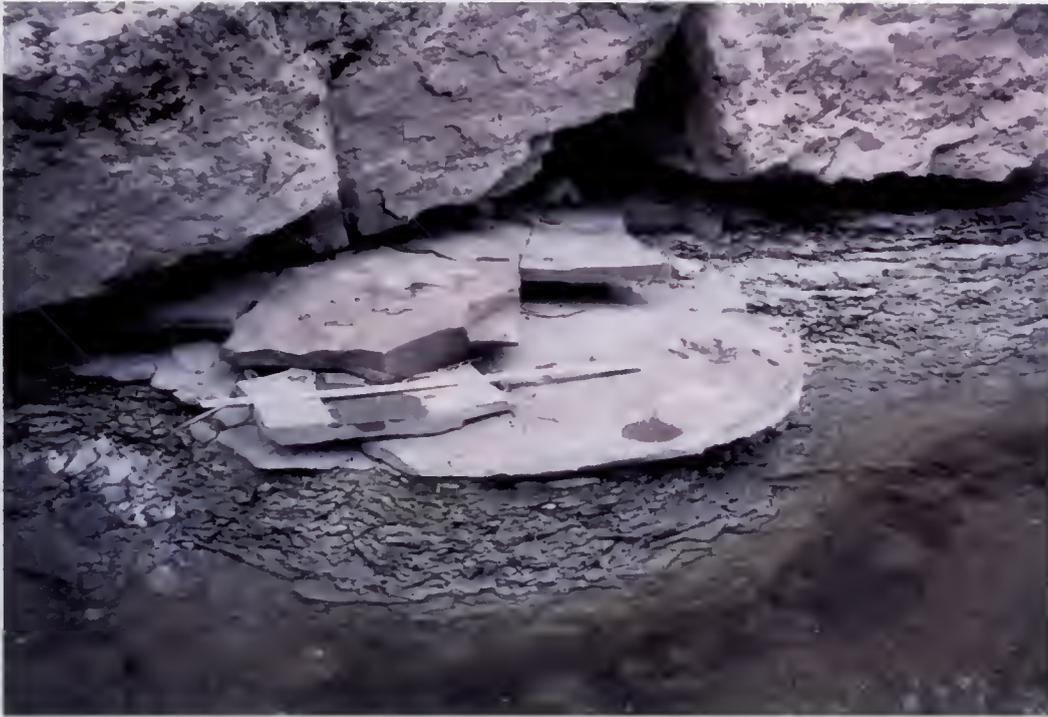
**Figure 3.1** Cooksville Creek, Mississauga, Ontario. The streambed is composed of weak shale and it can be seen that underneath the armourstones that the shale has been eroded and large gaps are present
