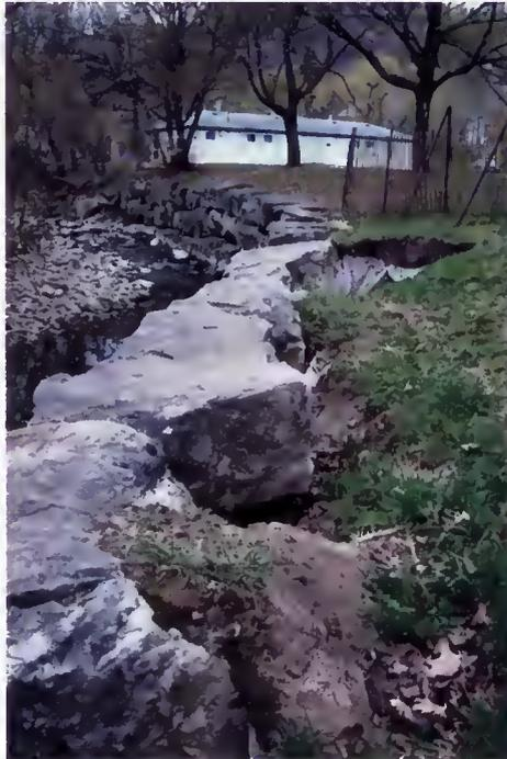
**Figure 3.22** Armourstone wall along Forty Mile Creek in Grimsby, Ontario before it was restored. Large depressions were noticed in behind the top layer of stones where sediment had been removed.
