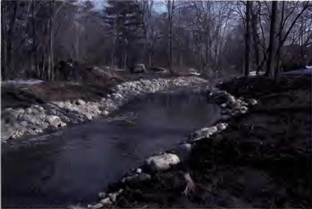
**Figure 2.3** Riprap lining a section of the bank along Loyalist Creek, Mississauga, Ontario. Photo is looking downstream. This picture was taken shortly after installation, February 2004.
