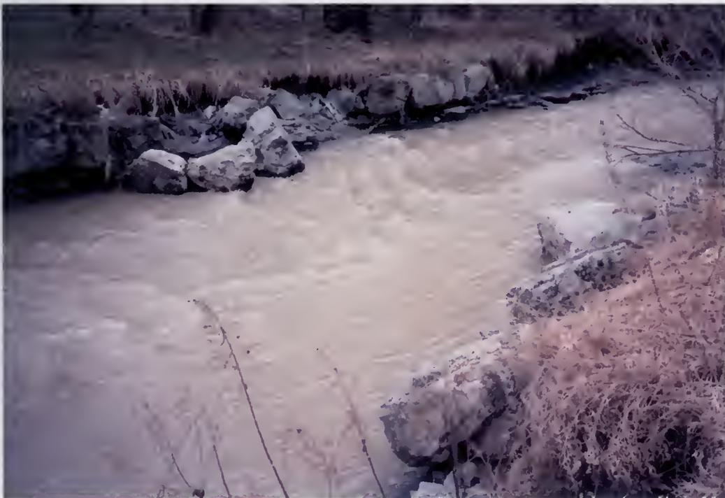
**Figure 3.2** Cooksville Creek, Mississauga, Ontario. This picture shows the collapse of the armourstone wall due to the removal of the shale which supports the armourstone. Photo was taken in 1997.
