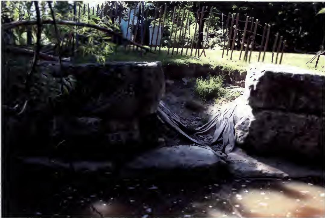
**Figure 3.3** Forty Mile Creek, Grimsby, Ontario. Two armourstones were removed from the wall and it can be seen that the base stone is still in tact and undermining has not occurred.
