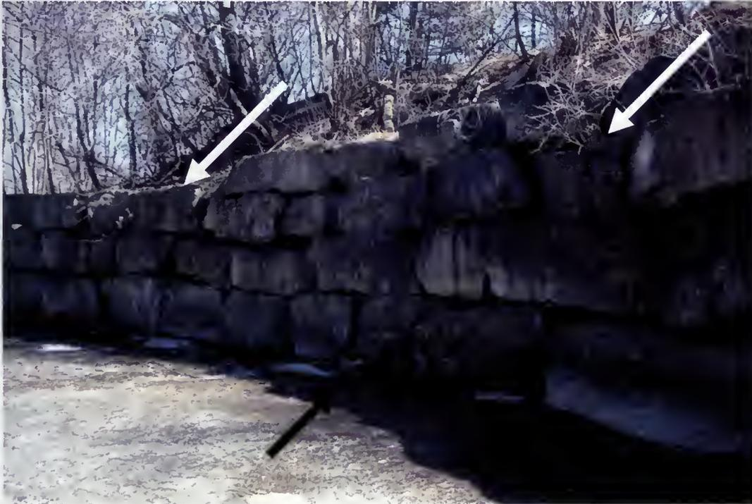
**Figure 3.9** Armourstone wall along Cooksville Creek near Aqua Drive, Mississauga, Ontario. Photo is looking downstream. Photo shows the transition from 4 stones to 3 (indicated by white arrows) and also shows the shale bed undercutting the stones (indicated by black arrow).
