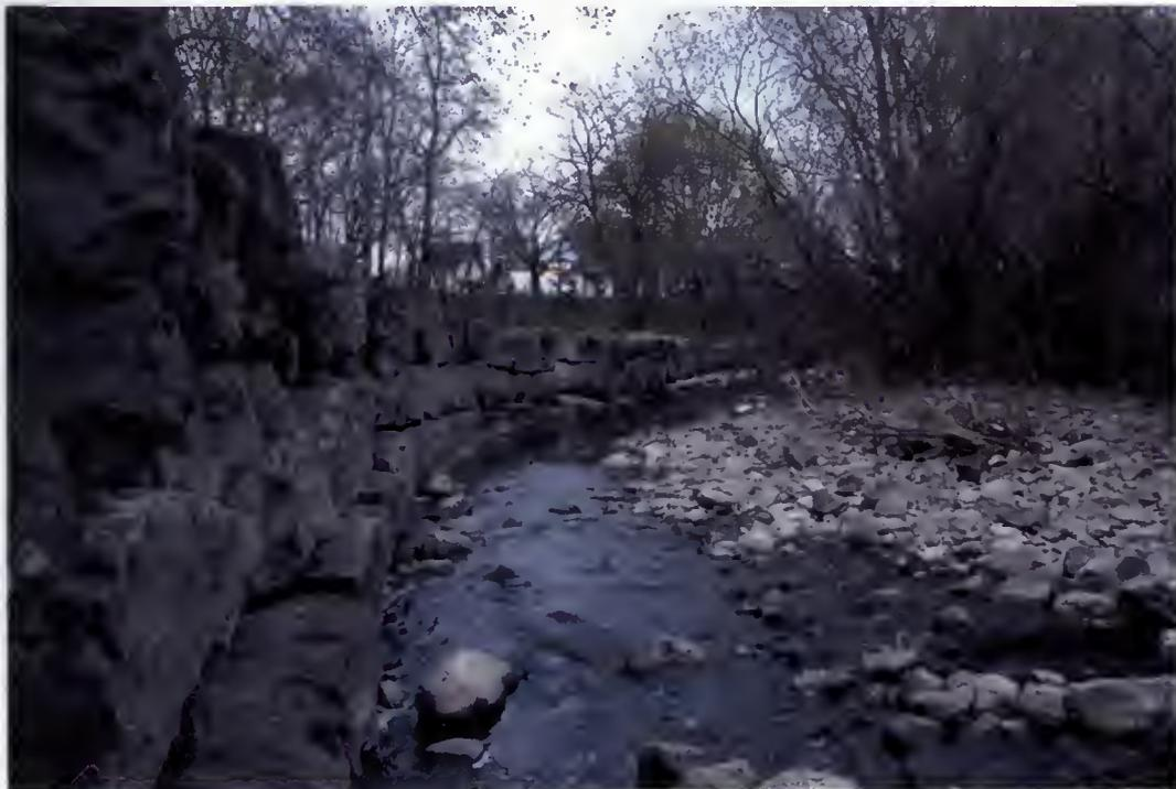
**Figure 2.4** Armourstone wall lining a section of the bank along Forty Mile Creek, Grimsby, Ontario. Photo is looking downstream. The armourstone wall is protecting adjacent parkland from erosion.
