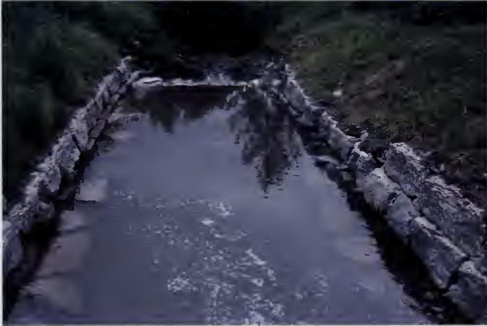
**Figure 6.5** Loyalist Creek Mississauga, Ontario. Armourstone blocks are placed on the streambed adjacent to the wall.
