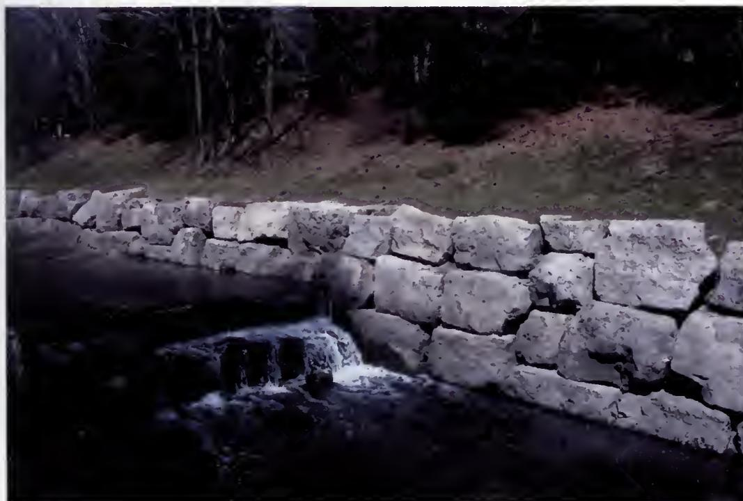
**Figure 3.7** Armourstone wall along Cooksville Creek near Robert Speck Parkway, Mississauga, Ontario. Armourstone walls are on both sides of the creek and this wall is located within an urban area.
