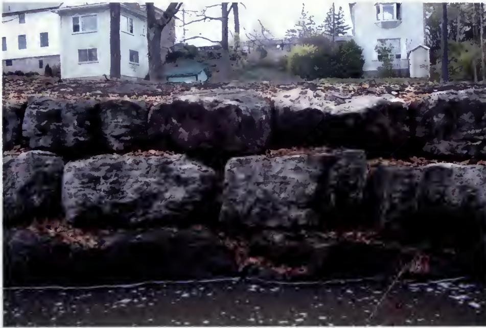
**Figure 6.1** Section of the armourstone wall along Forty Mile Creek, Grimsby, Ontario. This section shows how the stones can be staggered (as in a brick wall) so that they are resting on two stones below.
